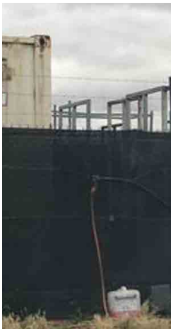
Figure 39 Example of effective border fence netting to contain EPS leakage
