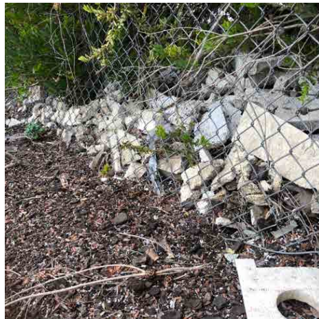
Figure 40 Example of border fence that does not contain proper netting
